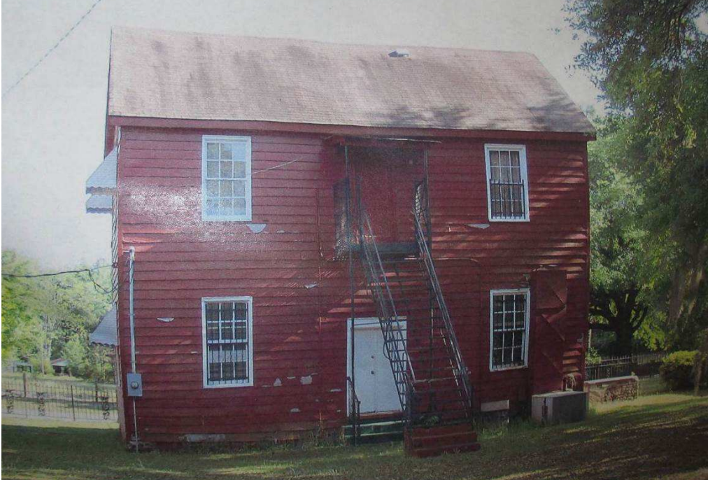
Figure 2.11 North (rear) elevation of St. James Schoolhouse c. 2011, before the 2011 addition was built. Most of this back wall was removed with the new addition. (Photo courtesy of St. James the Greater Parish.)
